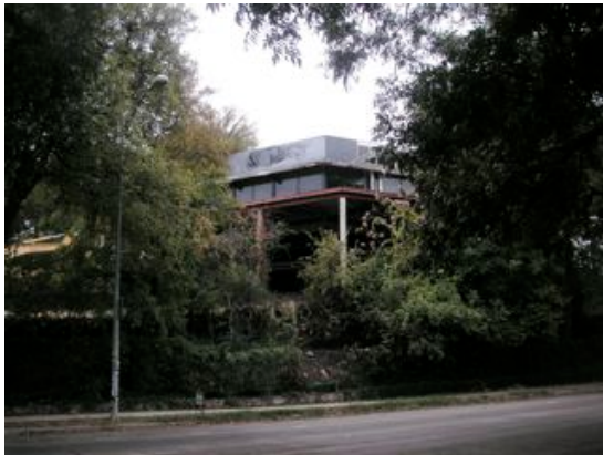
Just before demolition
